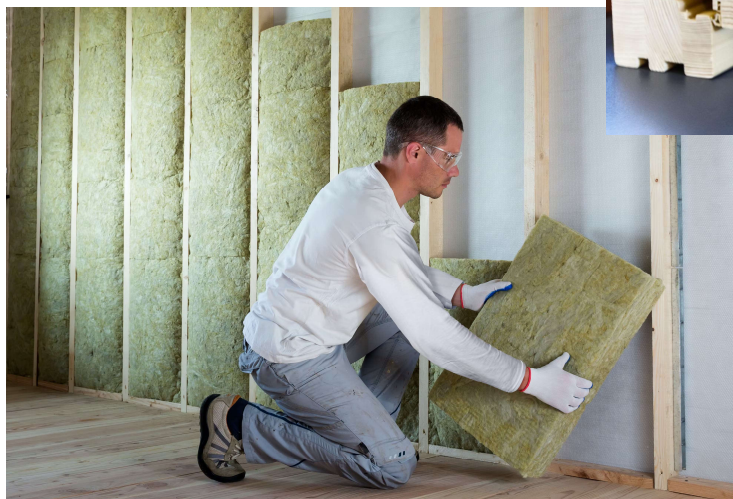
Internal Wall Insulation
